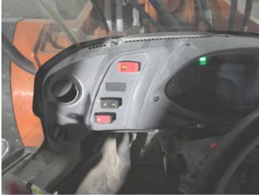
Switches and Controls
